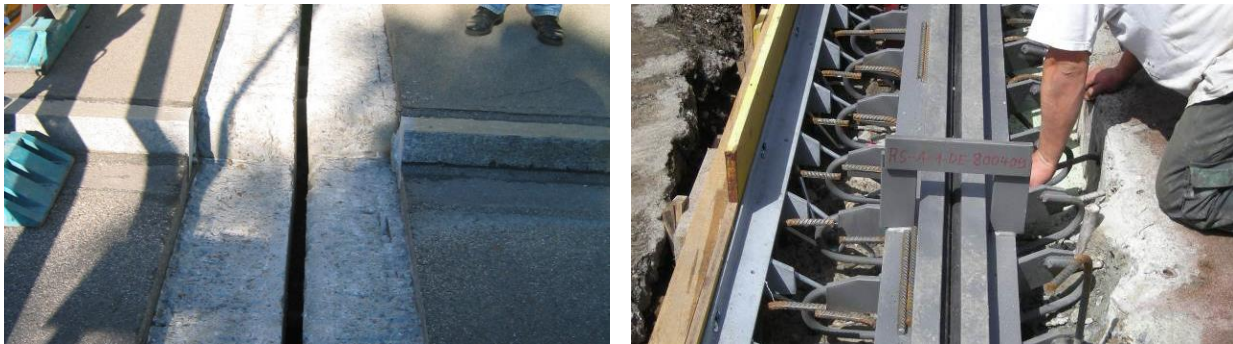
Figure 4: When installed on an existing structure to replace an old expansion joint, the anchorage in polymer concrete minimises break-out (often requiring only removal of the old joint and asphalt surfacing) (left) – far easier and less disruptive than a joint requiring anchorage in normal concrete (right)
