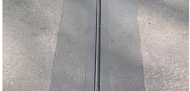
Figure 8: A “hump seal”, similar to the v-shaped seal shown in Figure 7 but featuring an additional hump which fills out the gap – keeping it clean, reducing noise under traffic and increasing pedestrian comfort
